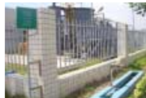
Wastewater treatment facility
