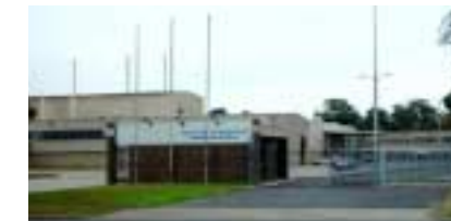
Rubber refining plant (Minto Plant)
