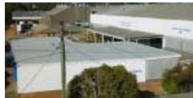
Anti-vibration rubber plant (Enfield Plant)
