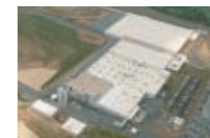
Full implementation of production at our tire plant in North America (Toyo Tire North America Manufacturing Inc.)
