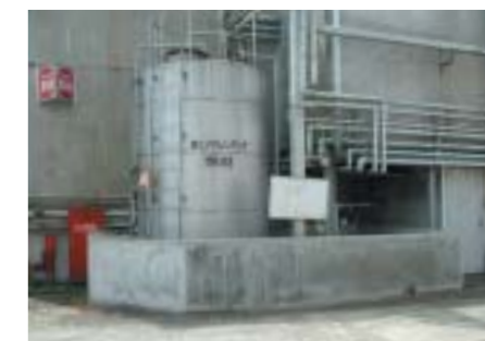
Dike for an outdoor chemical tank
