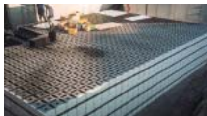
A rainwater storage permeation system built using the TUTT method
