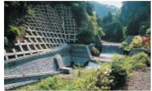
Harmony with local scenery and the use of recycled materials are key priorities for projects in Gifu Prefecture. Environmental colors have been used throughout this river improvement project, the aim of which is to prevent erosion and provide a path for fish. (Hachiman, Gujo-gun, Gifu Prefecture)
