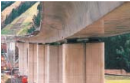
Rubber bearings enhance the earthquake resistance of bridges.
