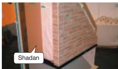
Cross-sectional structure of a building in which the Shadan system has been used.
