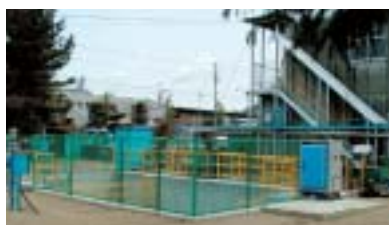
No. 1 Oil-Water Separation Tank after completion of upgrade
