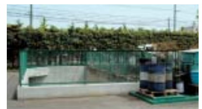
No. 2 Oil-Water Separation Tank after completion of upgrade
