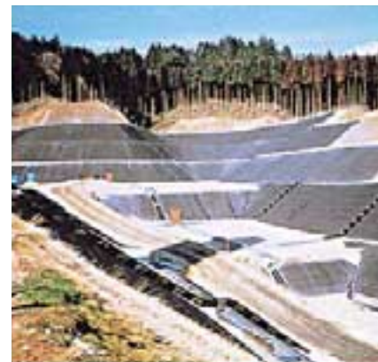
Shielding sheet-laying work
