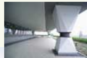
Seismic isolation installed in the garden terrace section on the third floor (top), and exterior of the Center building (left)
