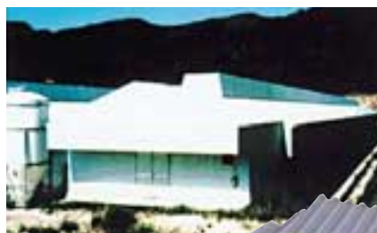
A barn built with Toyo Galdan, and thermal-insulating boards in various shapes
